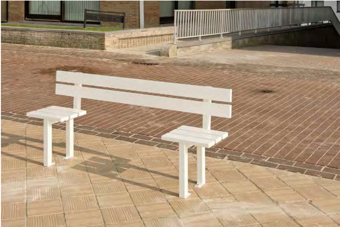
the center of the bench's seat has been removed
